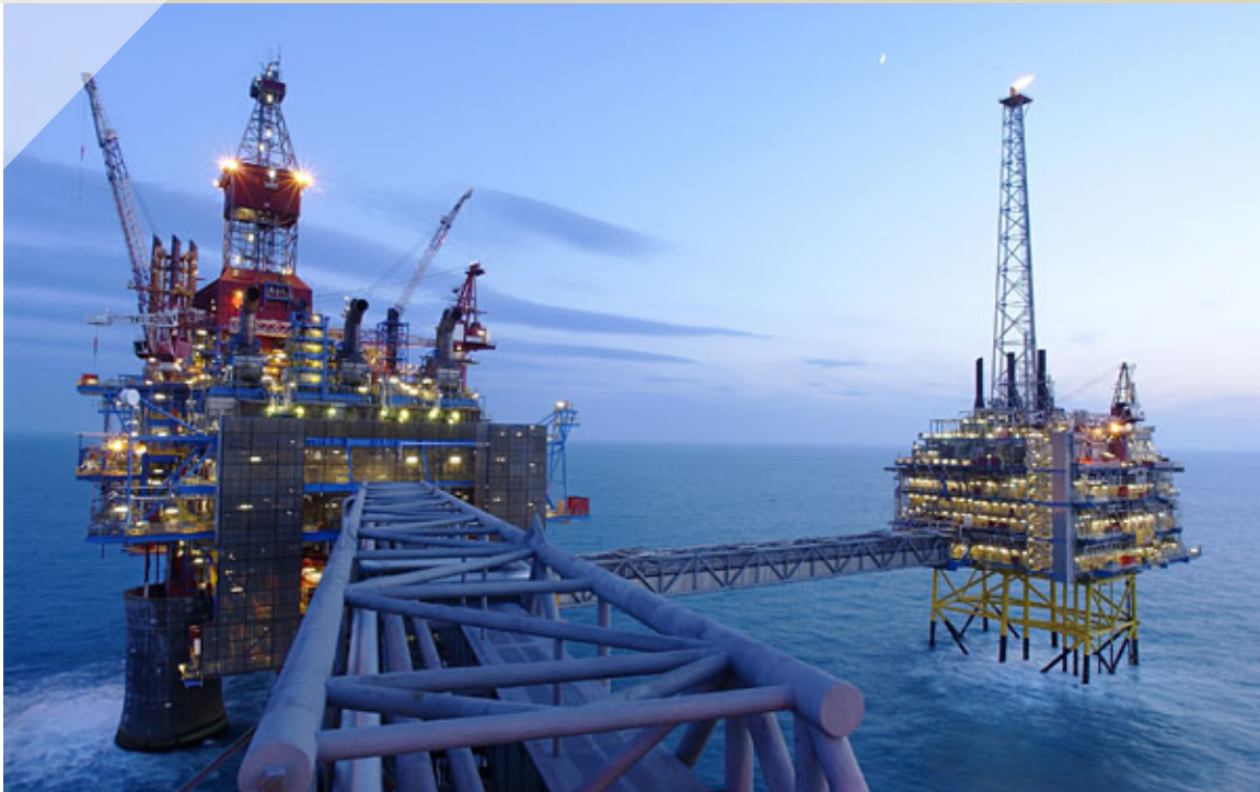
The Sleipner. A project that injects carbon dioxide into saltwater aquifers deep beneath the sea floor off the Norwegian coast [source: Stanford University].
